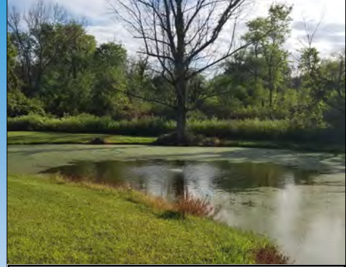
A stormwater pond with excessive vegetation due to the lack of a vegetative buffer
