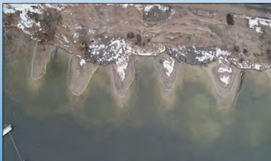
Note how far the road is from water on new shoreline
