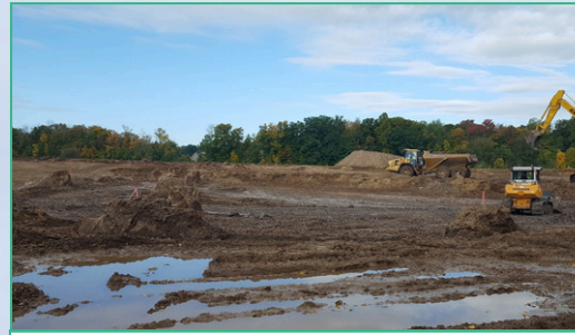
Start of grading, digging, and hauling of soil to create the first cell of the pond
