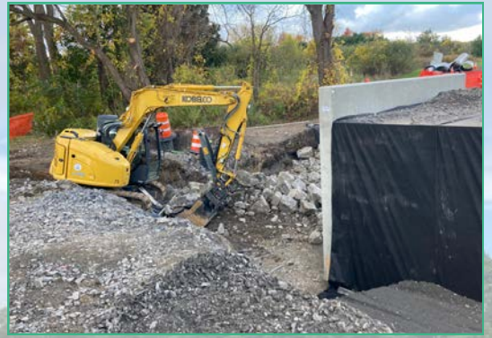
Start of grading, digging, and hauling of soil to create the first cell of the pond
