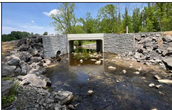
Above: Completed offline stormwater basin that will receive stormwater overflows from Shipbuilders Creek Below (L): Completed culvert over Shipbuilders Creek with inflow structure to send overflows to the facility Below (R): Completed outlet from Shipbuilders Creek into the facility
