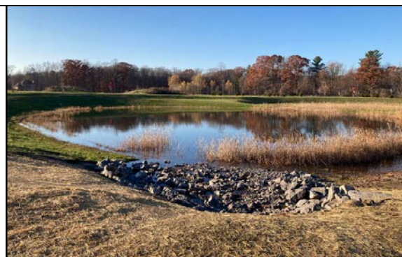
Above: Completed offline stormwater basin that will receive stormwater overflows from Shipbuilders Creek Below (L): Completed culvert over Shipbuilders Creek with inflow structure to send overflows to the facility Below (R): Completed outlet from Shipbuilders Creek into the facility
