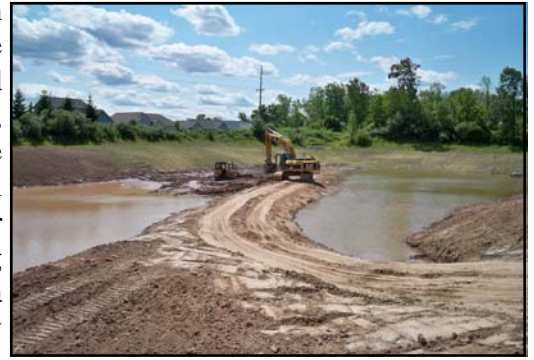
The Webster pond during construction.
