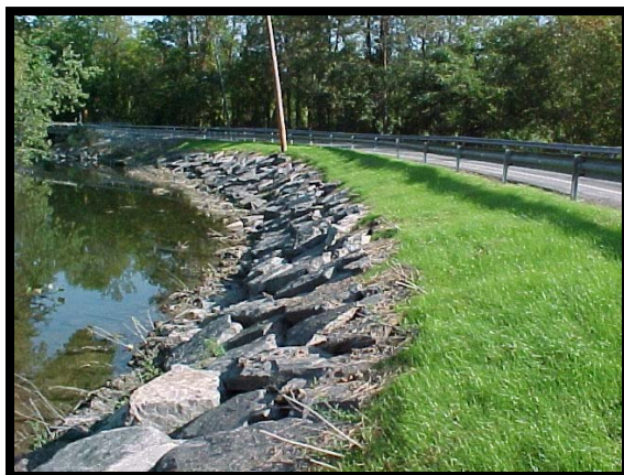
Stottle Road Stabilization.
