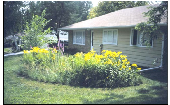
The rain garden allows roof runoff to soak into the ground through an engineered soil media. It is an attractive, aesthetically pleasing garden bringing color and microhabitat to a landowner's yard. (Photo: DEC)
