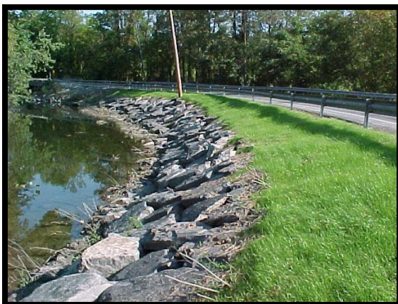
Stottle Road Stabilization.
